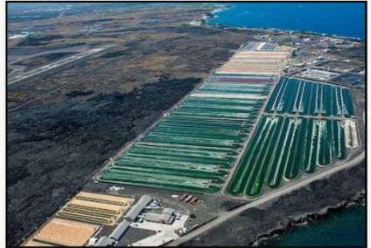
Microalgae cultivation facility provides a sustainable approach to wastewater treatment and management.
